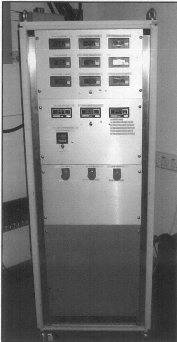
(a) Data acquisition cabinet
