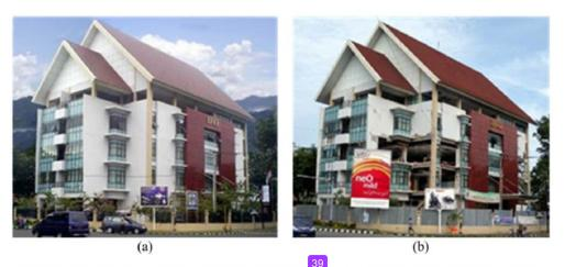
Figure 2. Views of the BPKP building before and after the earthquake. (a) Before the earthquake. (b) After the earthquake.
