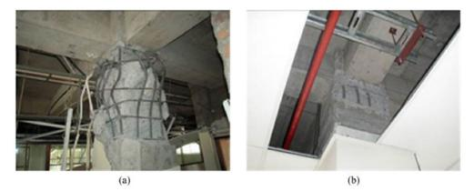
Figure 4. Significant damage to the third-story columns. (a) Damage class V (X5–Y4). (b) Damage class IV (X5–Y2).
