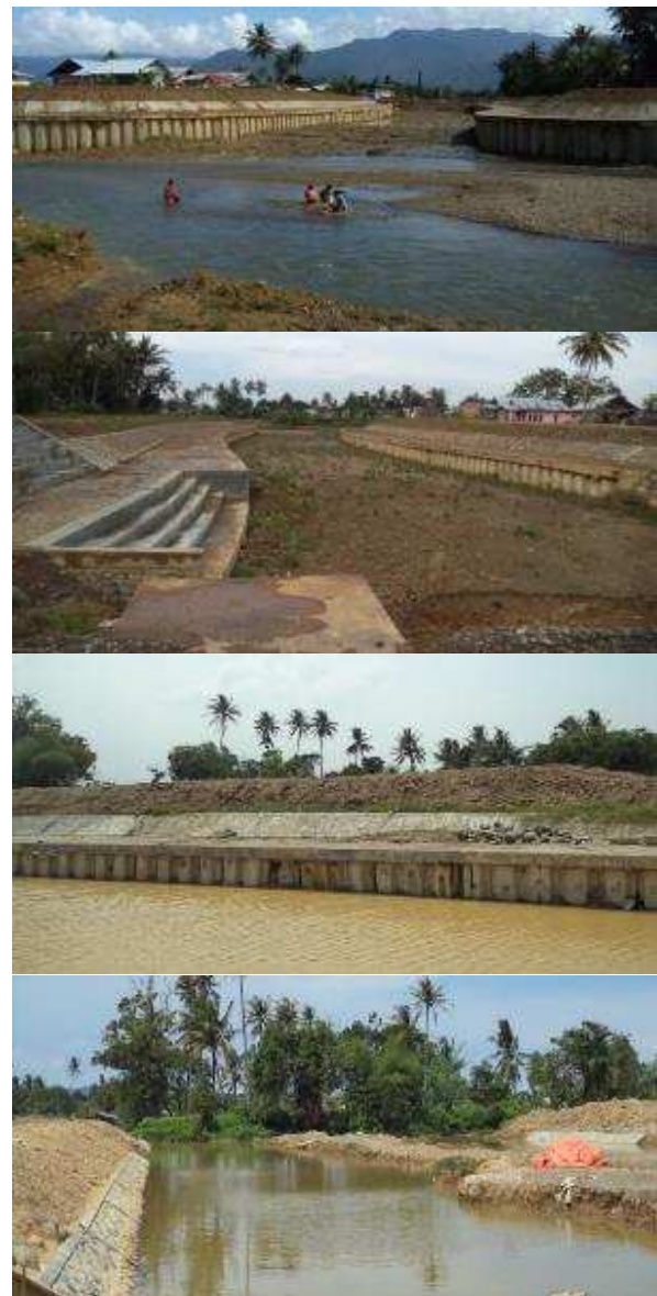
Figure 4. Luruih River normalisation project (source: Dinas PSDA Sumbar)
