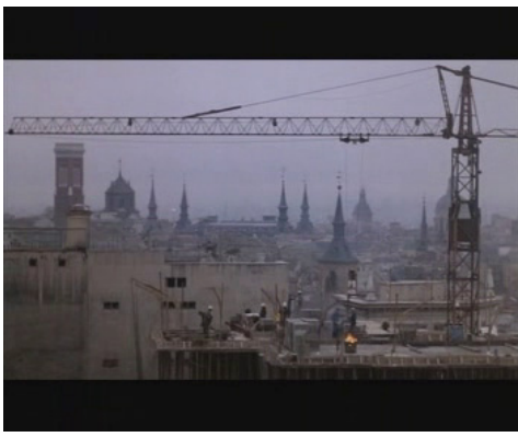
Fig. 10: Cranes take over the Madrid centre in El Crack II .
