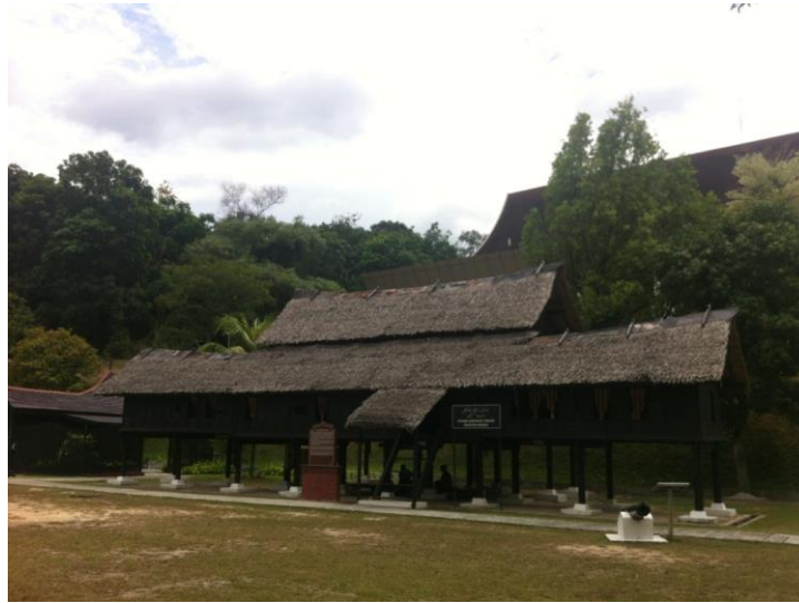
Figure 5: Façade of Istana Ampang Tinggi, Negeri Sembilan
