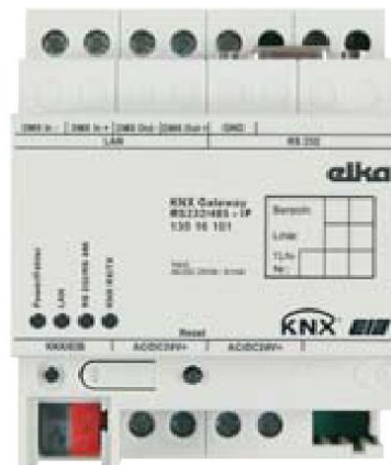
Figura 31. Interfaz KNX-RS232/485-IP
