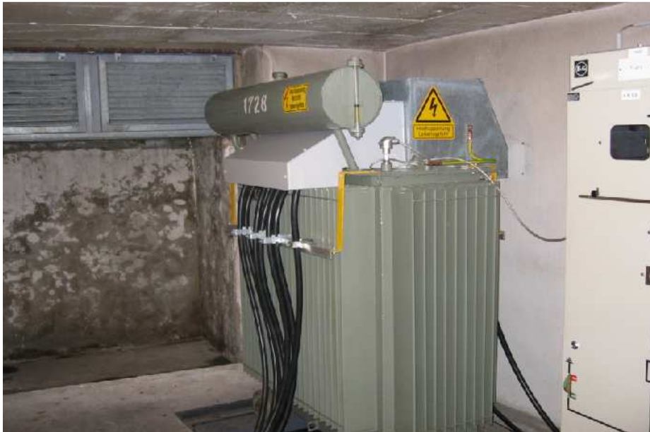
Figure 33: “MV/LV TRANSFORMER”
