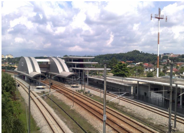
Figure 3.5: The ERL KLIA Transit Station
