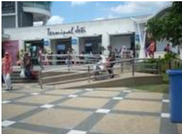
Figure 3.12: Ramp leading into the Terminal
