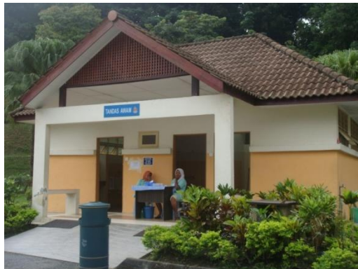
Figure 4.18: Income for maintaining facilities
