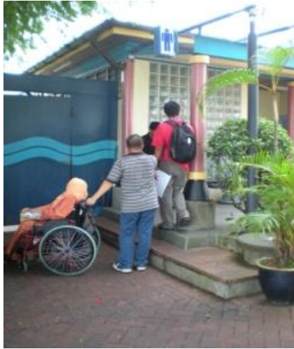
Figure 6.11: Steps leading to the public toilet
