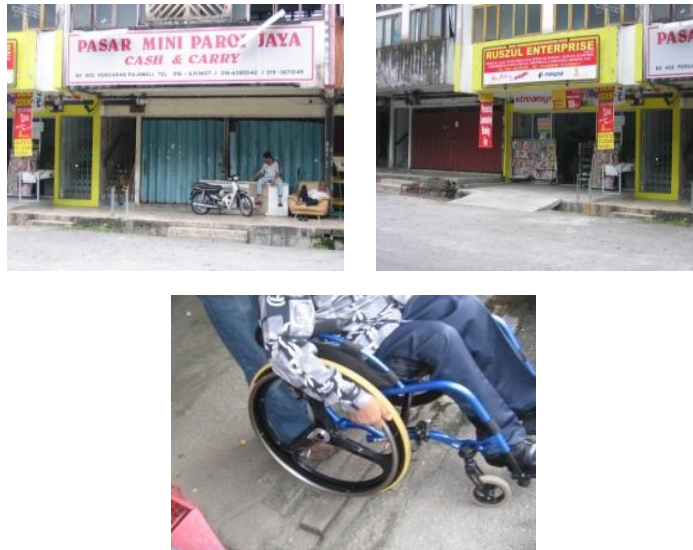
Figure 5.14: Changes of leveling among shops and bumpy surface to the shop corridor.
