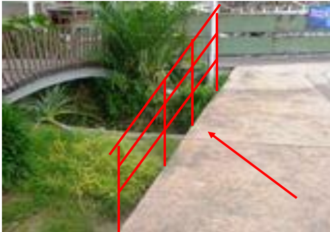
Figure 6.4: The part of the promenade which is not provided with railings that separate the path and the open drain
