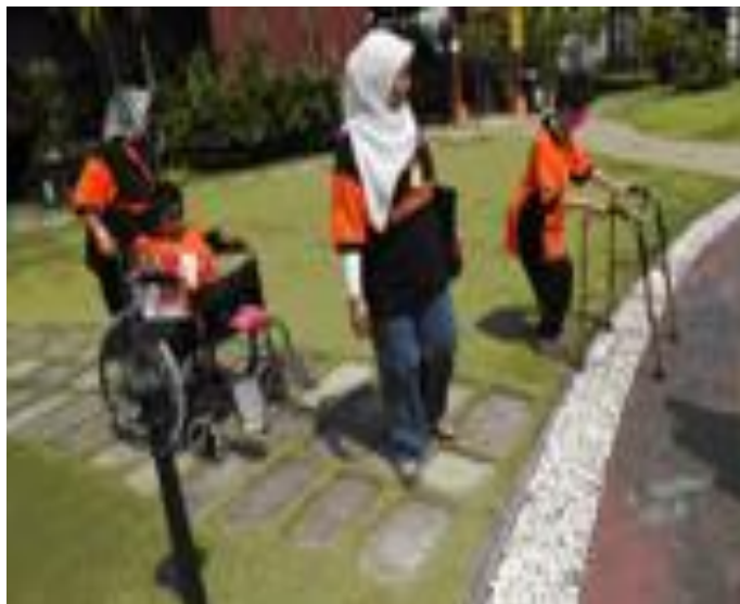
Figure 6.5: Inappropriate paving materials that limits access
