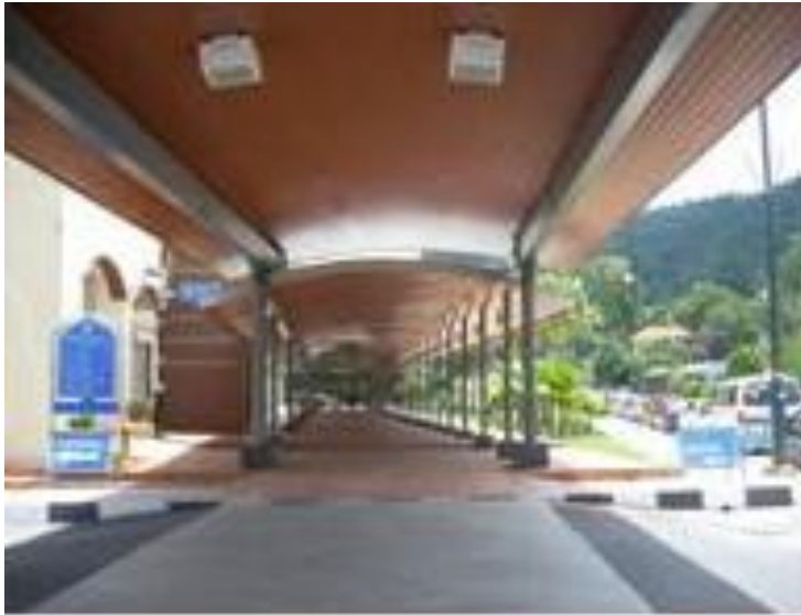
Figure 3.13: Covered corridor from car park
