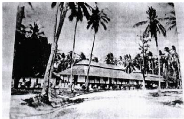
Figure. 1 An image of the single storey colonial hospital architecture of a tropical hospital in the garden. (Source: Balik Pulau Hospital, Penang website)
