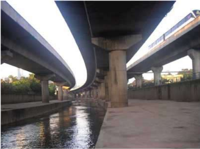
Figure 2. The construction of a highway and light railway transforming the Klang River in kampung Datuk Keramat as a longkang besar. Photograph by Nor Azlin.
