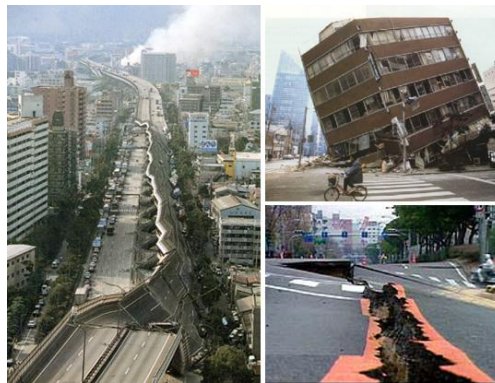
Photo.1 Kobe, Japan earthquake (1995).
