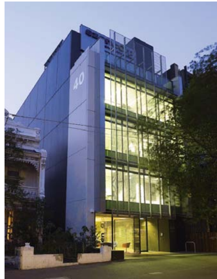
Zencorp 40 Albert Road South Melbourne Architect: SBP ESD: Aurecon and ECS 6 star Greenstar Office Design 5 star NABERS Energy 5 star NABERS Water
