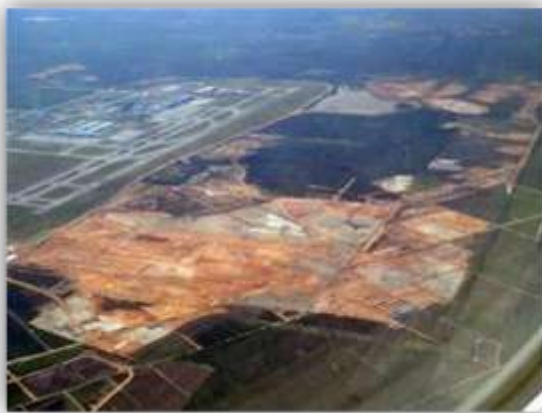
Figure 5: Construction underway at the site (KLIA 2)
