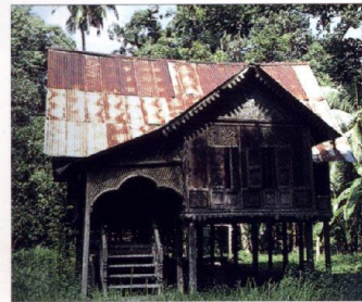
Building materials with low thermal qualities, such as woven bamboo for walls and thatch for roofs (above), have been largely replaced by timber and galvanized iron (below).
