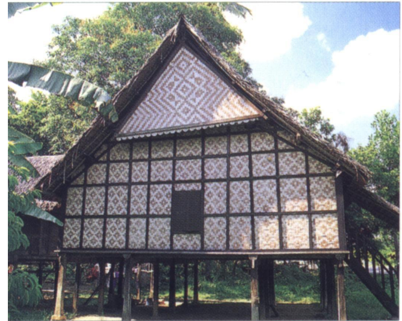
The bamboo walls and atap roof of the rumah kutai in the Kuala Kangsar district of Perak allow natural ventilation and reduce glare.
