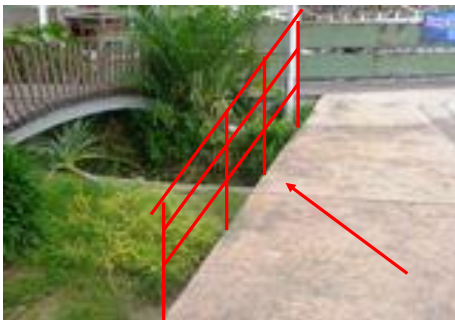
Figure 4: The part of the promenade which is not provided with railings that separate the path and the open drain
