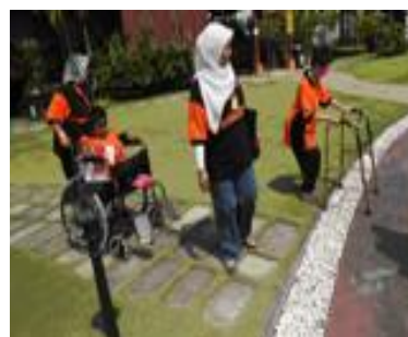
Figure 5: Inappropriate paving materials that limits access
