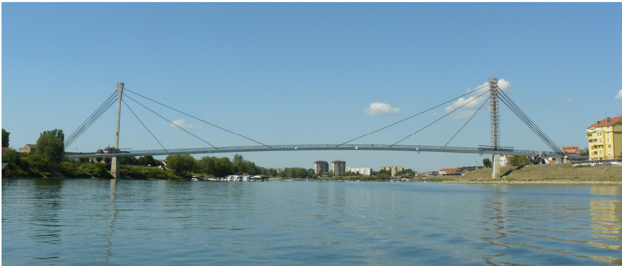
Figure 5: Pedestrian bridge in Sremska Mitrovica across the river Sava – downstream view
