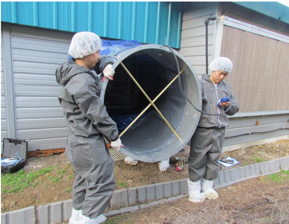
Fig. 10 Measuring air flow of sidewall fan
