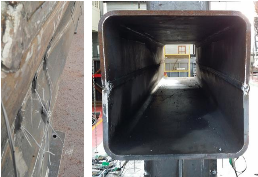
Figure 3.15 The chord sidewall indented at the mid-height of the specimen (X90-325-1.000-26.7)
