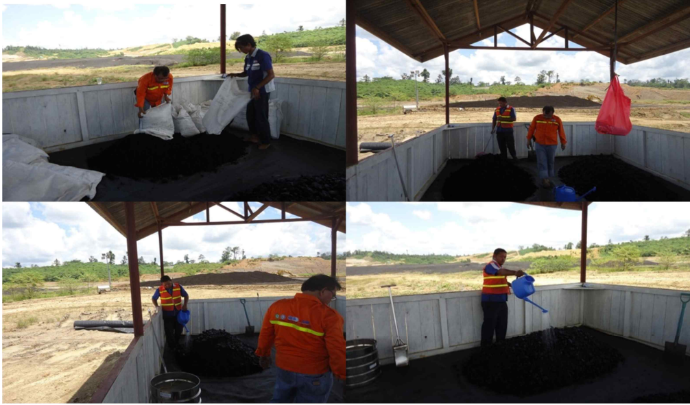
Fig 2-5 Air Drying Test under Roof
