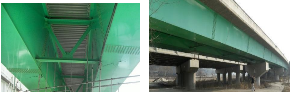
Figure 4. 1 Yeondae Bridge (Kim, 2014)
