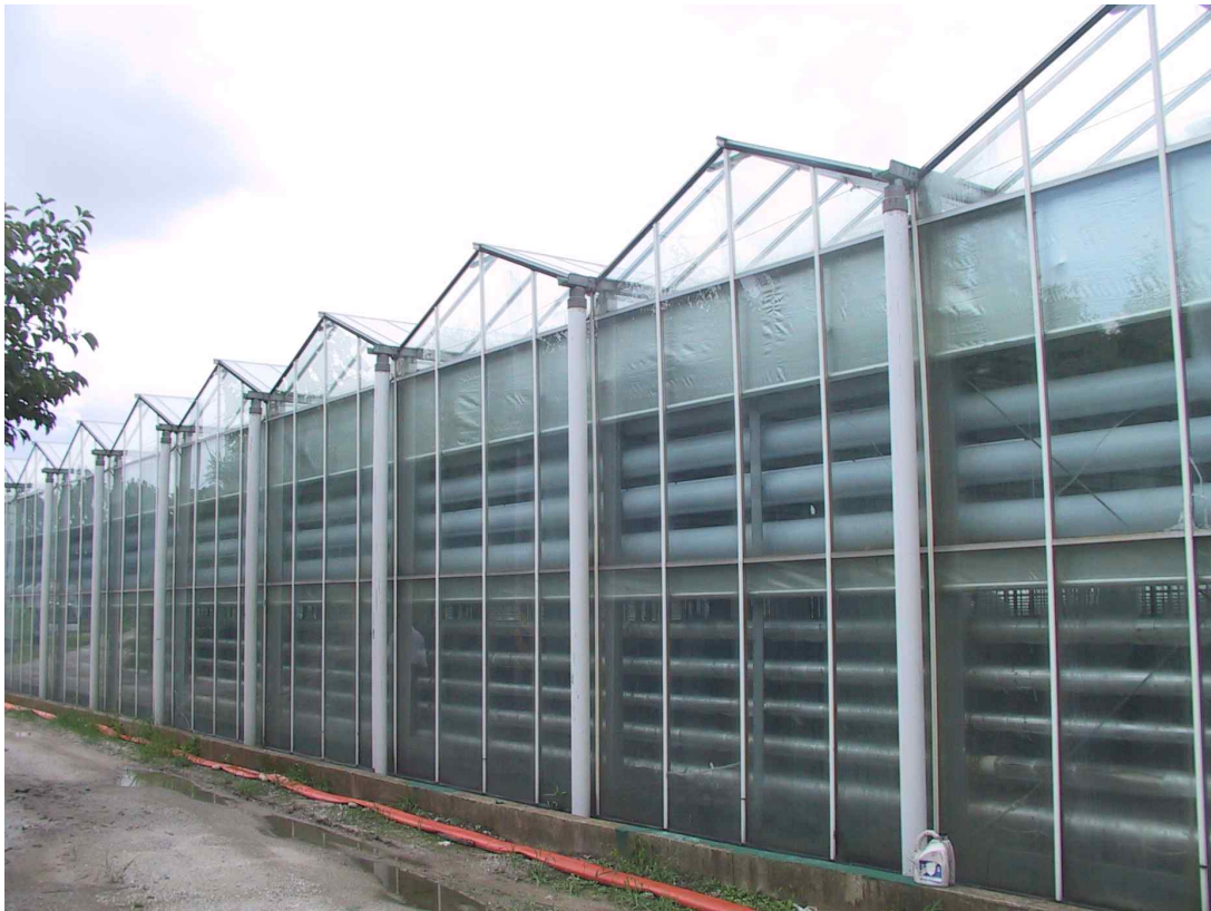
Fig. 6 17-span venlo-type greenhouse using geothermal energy system in Namwon used for this study
