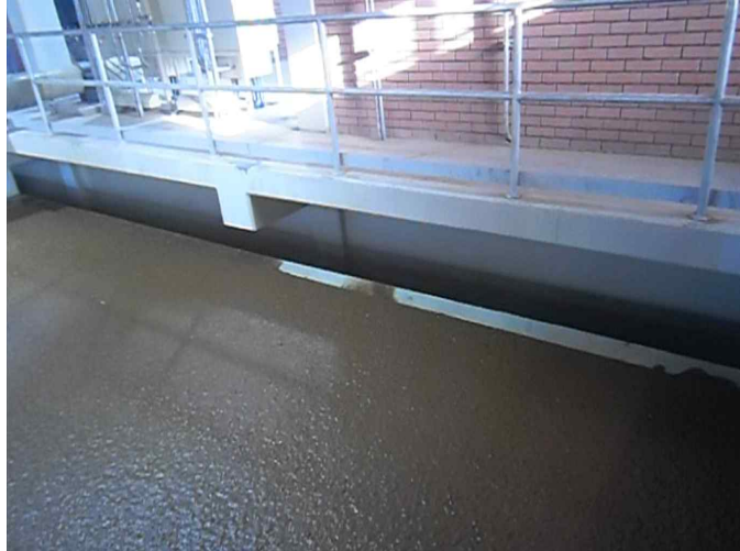
Fig. 2.5 Hydraulic float removal system
