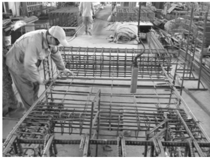
(a) Arrangement re-bar
