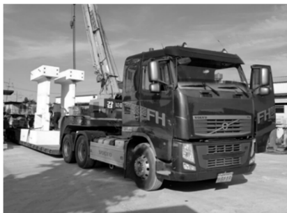
(f) Specimens lifting
