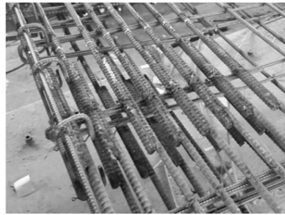
(b) U-shaped stirrups welding
