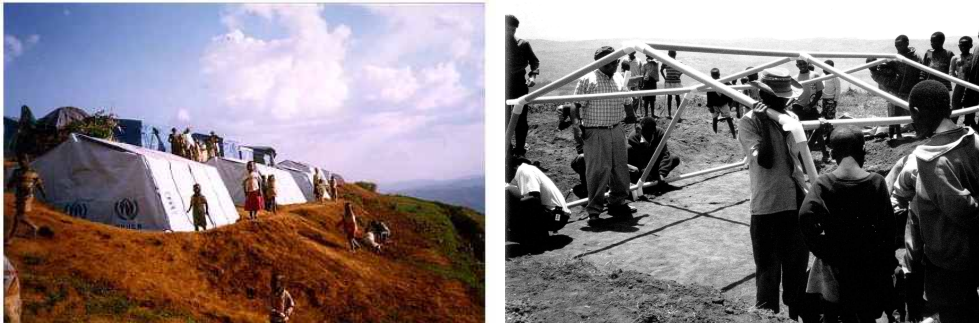
[그림 3-8] Paper Emergency Shelters for UNHCR (Rwanda, 1999) (출처: Ban, S., Miyake, R., (2009). Shigeru Ban: Paper in Architecture)
