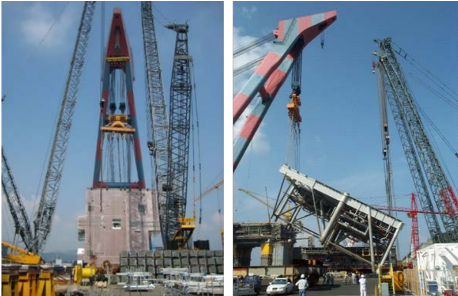
Figure 1-1 Block turn-over using 1 floating crane and 2 crawler cranes
