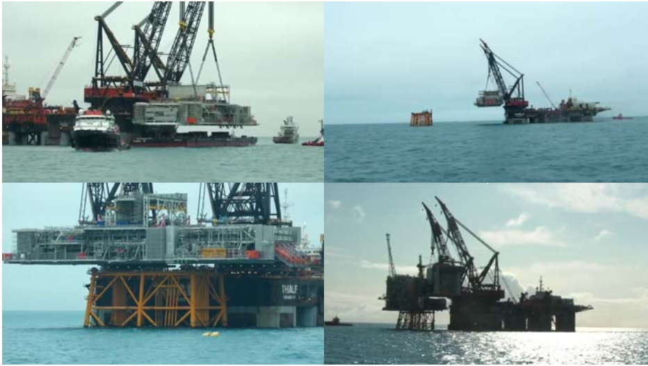
Figure 1-3 Topside module installation using dual crane rig and barge ship
