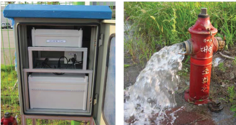
(b) Measurement station and water discharge
