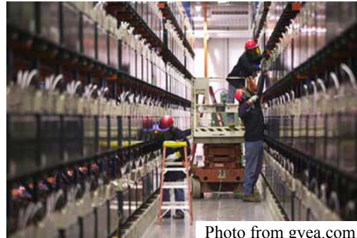
(b) Golden Valley Electric Association EES system, Fairbanks, AK, a 27 MW NiCd battery EES system for power grid
