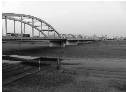
Fig 17. Akekawa River bridge
