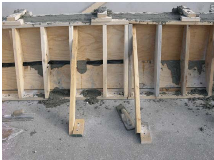
Figure 10. Permanent New Jersey Safety Shape Barrier System Construction
