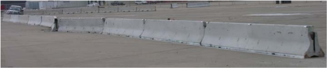
Figure 25. System Damage, Test NYTCB-4
