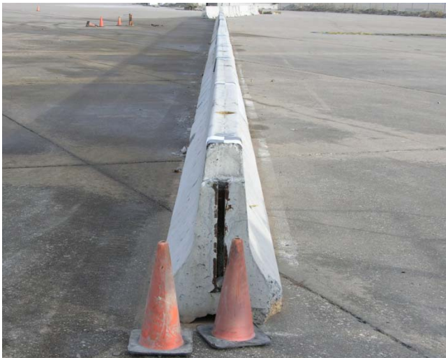
Figure 14. Pinned Temporary Concrete Barrier, Test NYTCB-4
