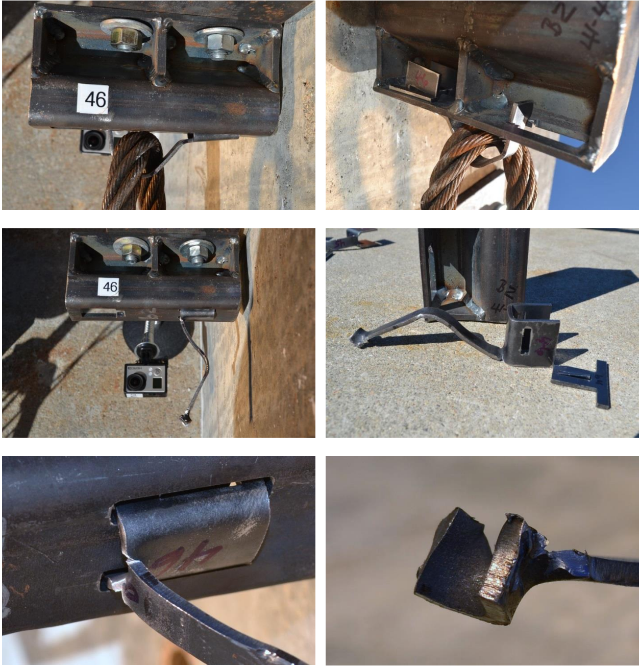
Figure 71. Pre-Test (Upper) and Post-Test (Lower) Photographs, Test No. HTTB-46
