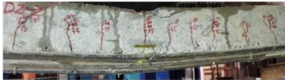
(e) Typical failure mode of Group D2
