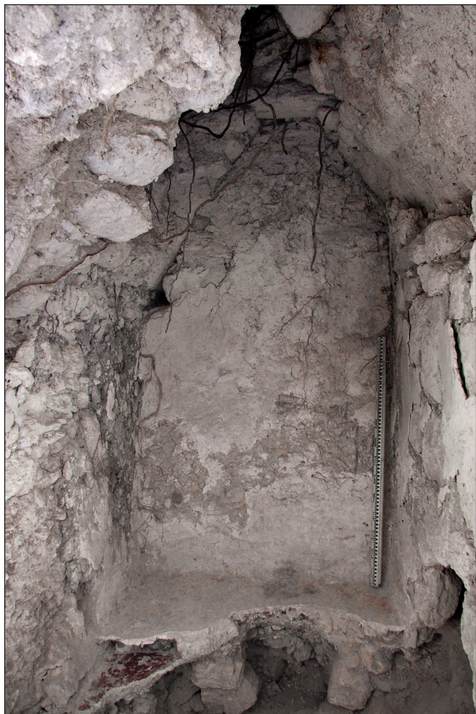
Figure 3. Photograph of the intact vaulted room of Str. TM-2, with its plastered walls and damaged portion of bench at the southern end of the room (photograph by Gail Hammond).
