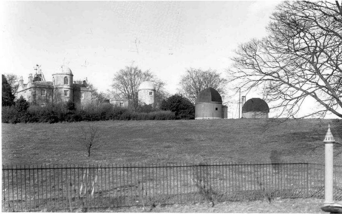
Plate 5. Armagh Observatory photographed from the southwest in 1930 showing the sunshine recorder on a steel tower to the left of the Calver Dome on the right
