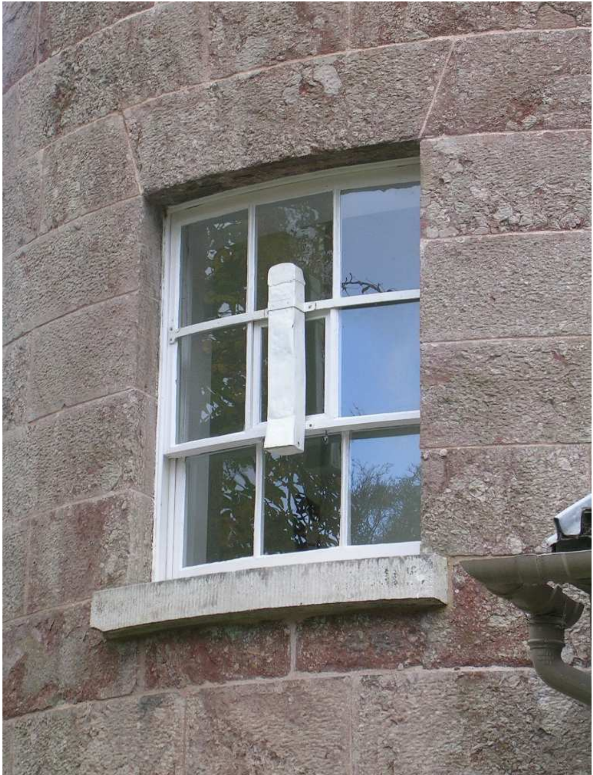
Figure 2. The bright metal box in the north window of the 1827 Tower which housed the external thermometer from 1834 and probably the wet and dry bulbs of the hygrometer from 1838 until the installation of the Stevenson Screen in 1885
