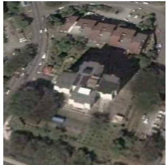
Figure 4.10: Satellite picture of building E
