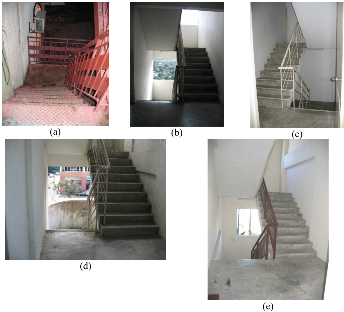
Figure 4.42: (a) Metal staircase, (b) Staircase with square opening, (c) Closed staircase, (d) Staircase with half round floor, (e) staircase with windows
