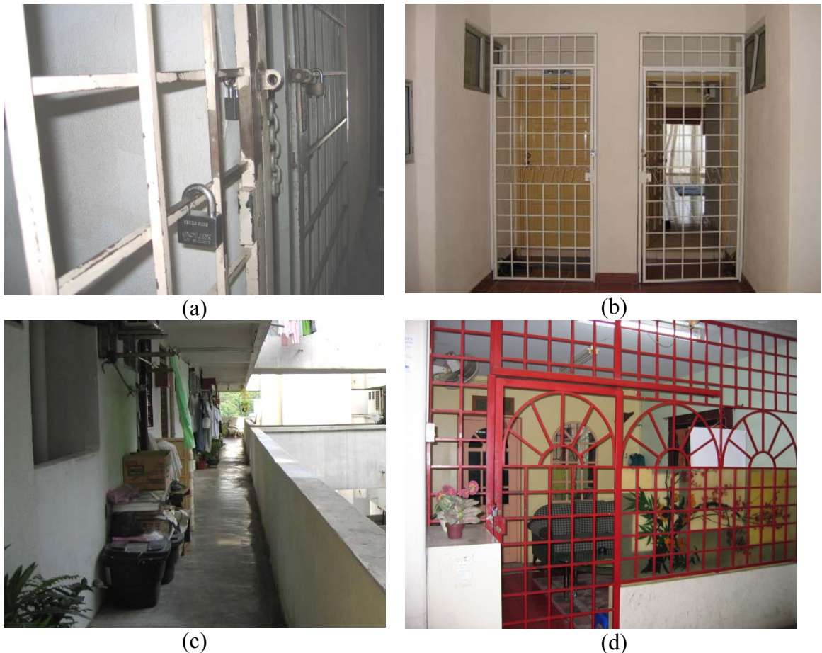
Figure 5.23: (a) Double lock iron grill, (b) Iron grill fitted at the main doors, (c) Items placed in corridor, (d) Iron grill built-up beyond the property limit.
