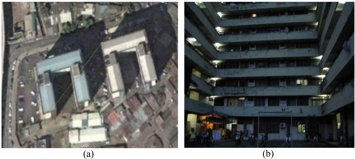
Figure 4.4: (a) Location of Building B, (b) Façade view of building B
