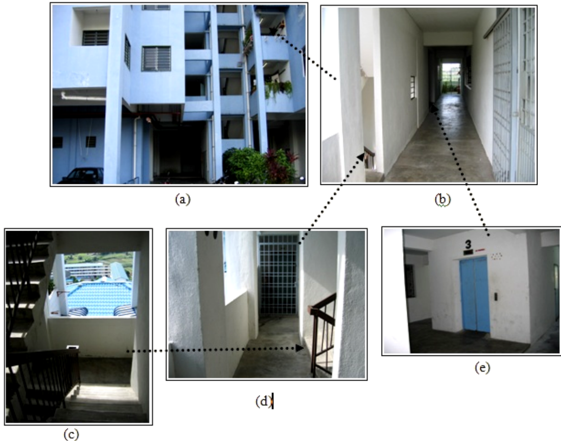
Figure 4.15: (a) View of building P2. Main entrance through passageway at ground floor besides the staircase shaft. (b) Corridor designed with access to both staircases and lifts. (c) Staircase designed parallel with corridor and having a wide opening for natural ventilation. (d) Staircase designed with access from both corridors (e) View the location of one of the lifts provided in this building. Another lift was located opposite the lift shown in this picture.
