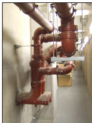
Drainage exit point from building
