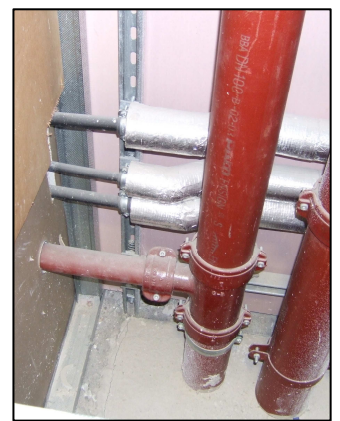
whb branch connection into stack
