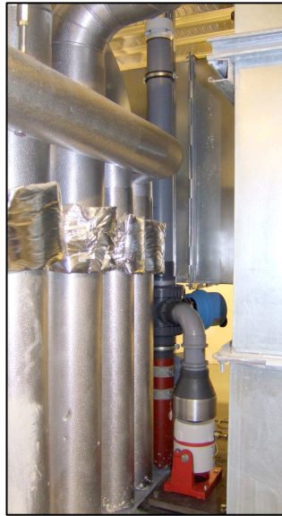
Transient entry device installed on Stack 2
