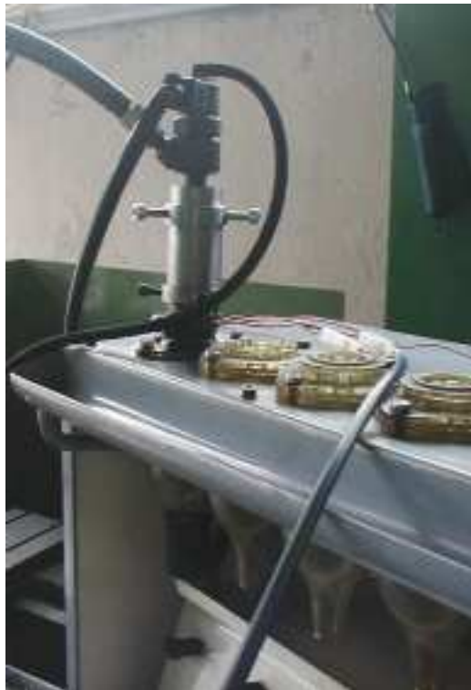
Figure 3.11: The nozzle metal port (prior to fitting the insulation).
