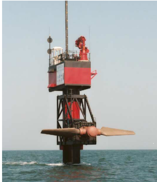
Figure 6.11: The Seaflow turbine, with blades raised for maintainence (courtesy of MCT website [1])
