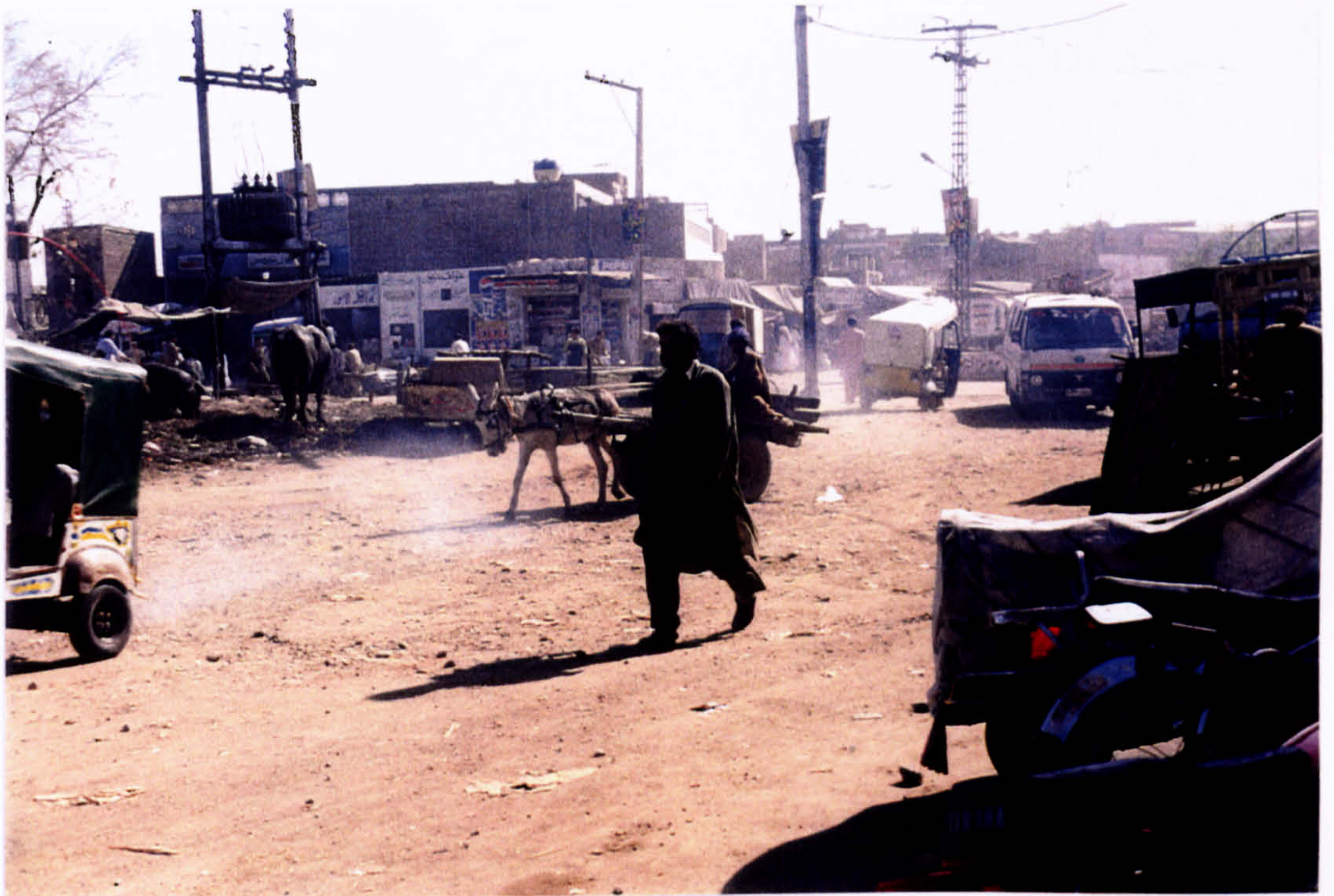
Plate 6.1a Dilapidated road conditions in Faisalabad
