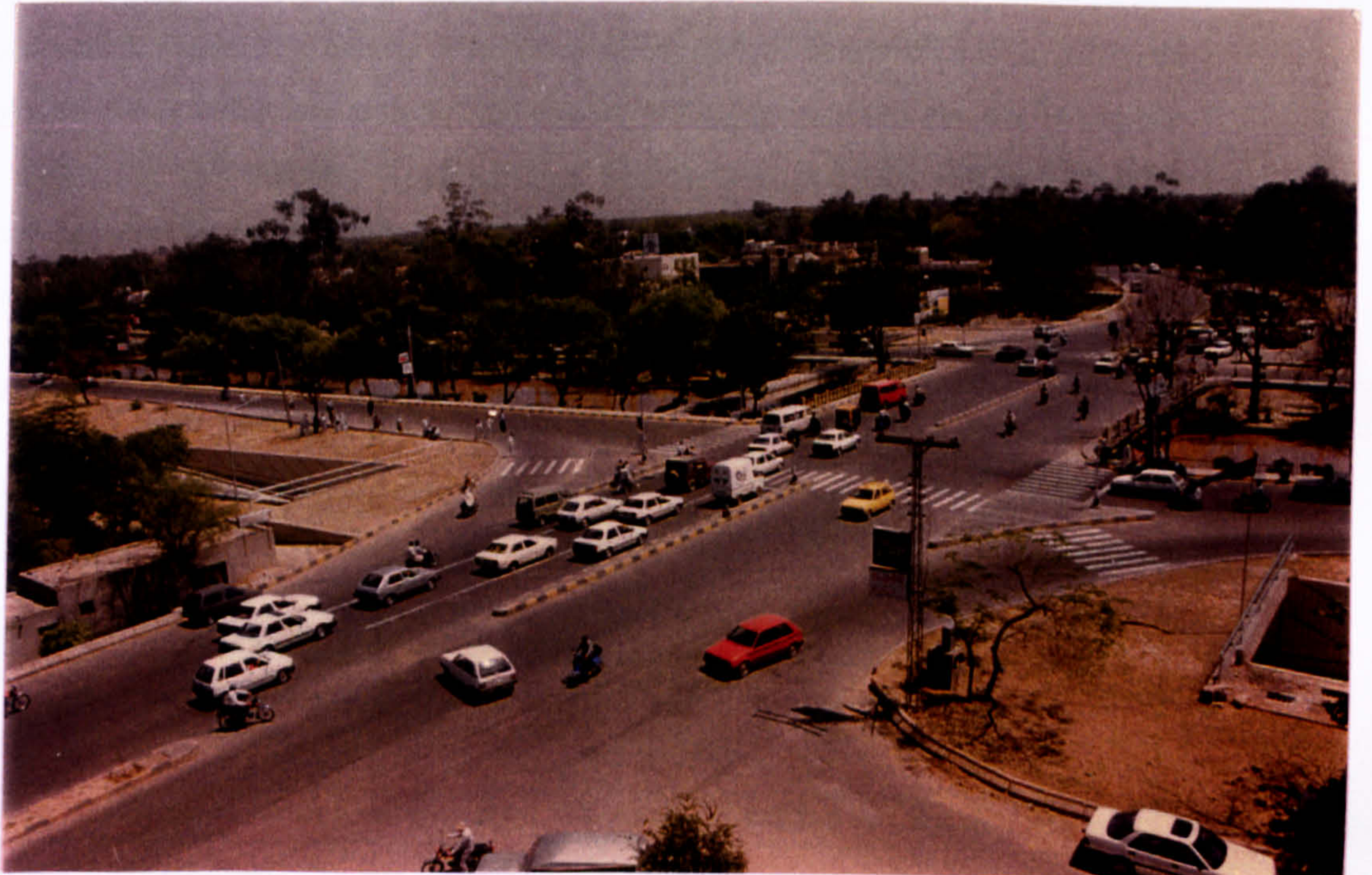
Plate 5.2 A newly built under pass on Jail Road in Lahore
