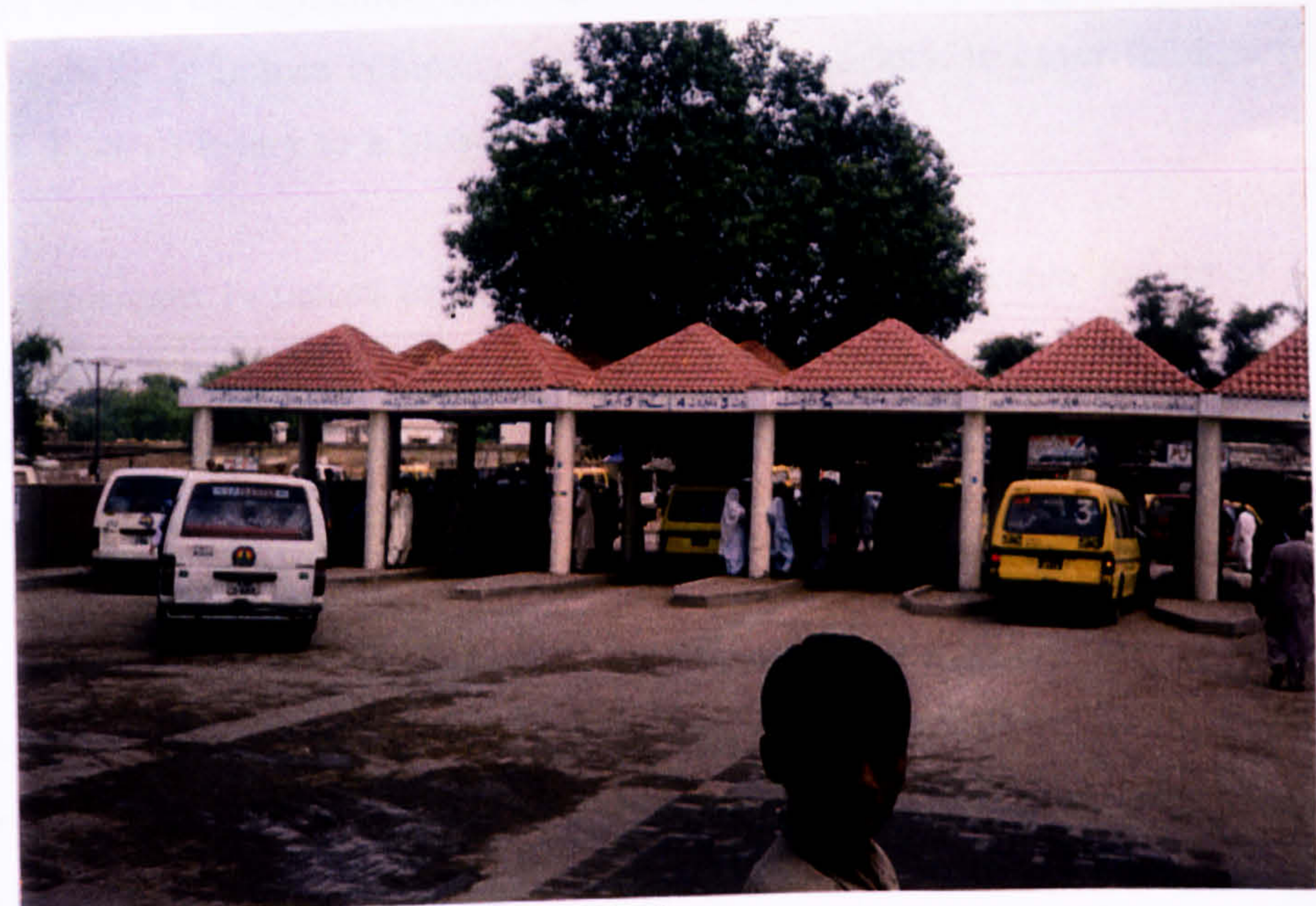
Plate 6.5 Well organised FUTS terminal
