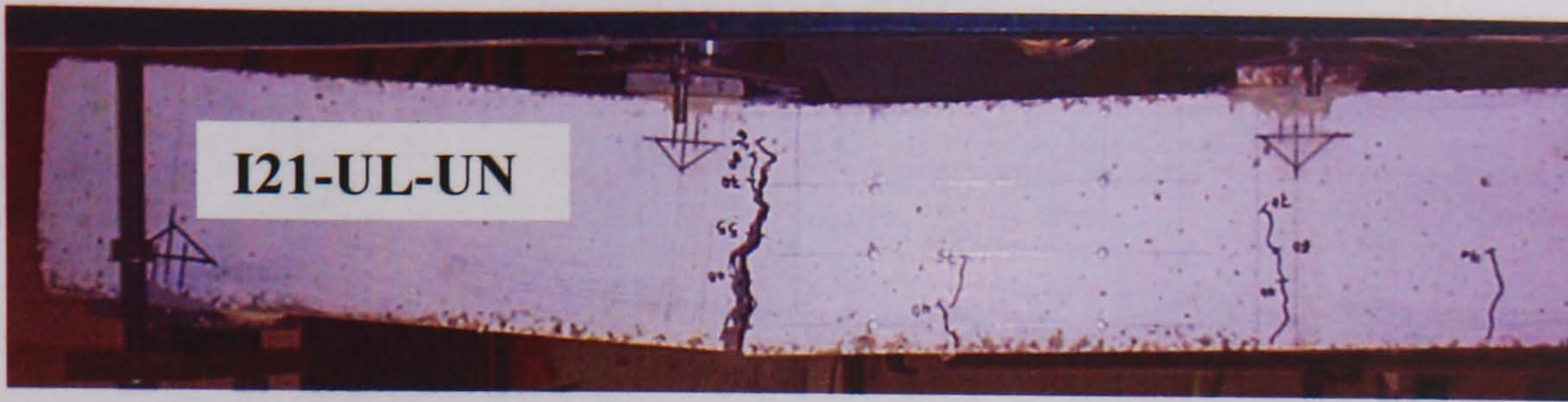
Figure 4.1: Typical flexural failure due to steel yielding near to the point load, beam I21-UL-UN
