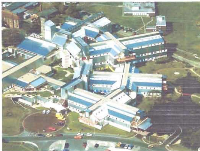
Figure 3: An Example of a Nucleus Prototype, St. Mary's Hospital in the Isle of Wight
