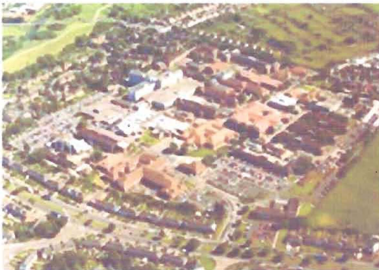
Figure 2: An Example of a Harness Prototype, East Birmingham Hospital in the West Midlands
