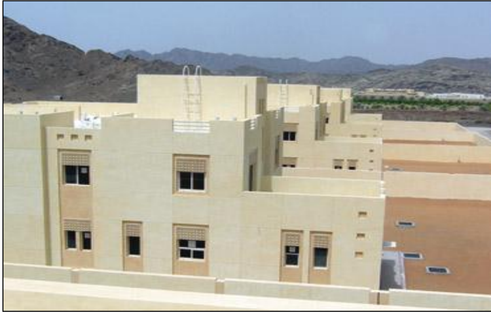
Figure 45: New houses for those people who affected by Earthquake 2002
