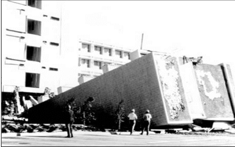
Figure 63: San Fernando, California earthquake 1971 (USGS 2007)
