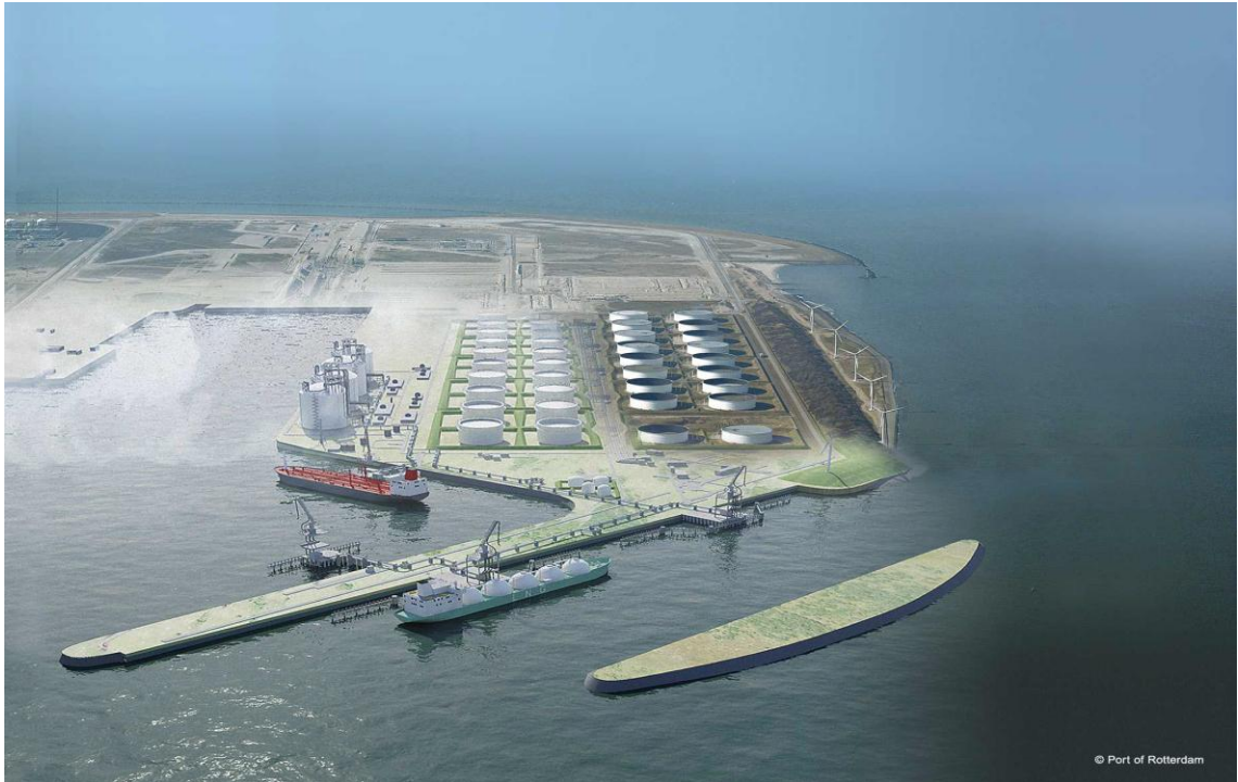
Figure 2.5 The Gate Terminal in the Netherlands
