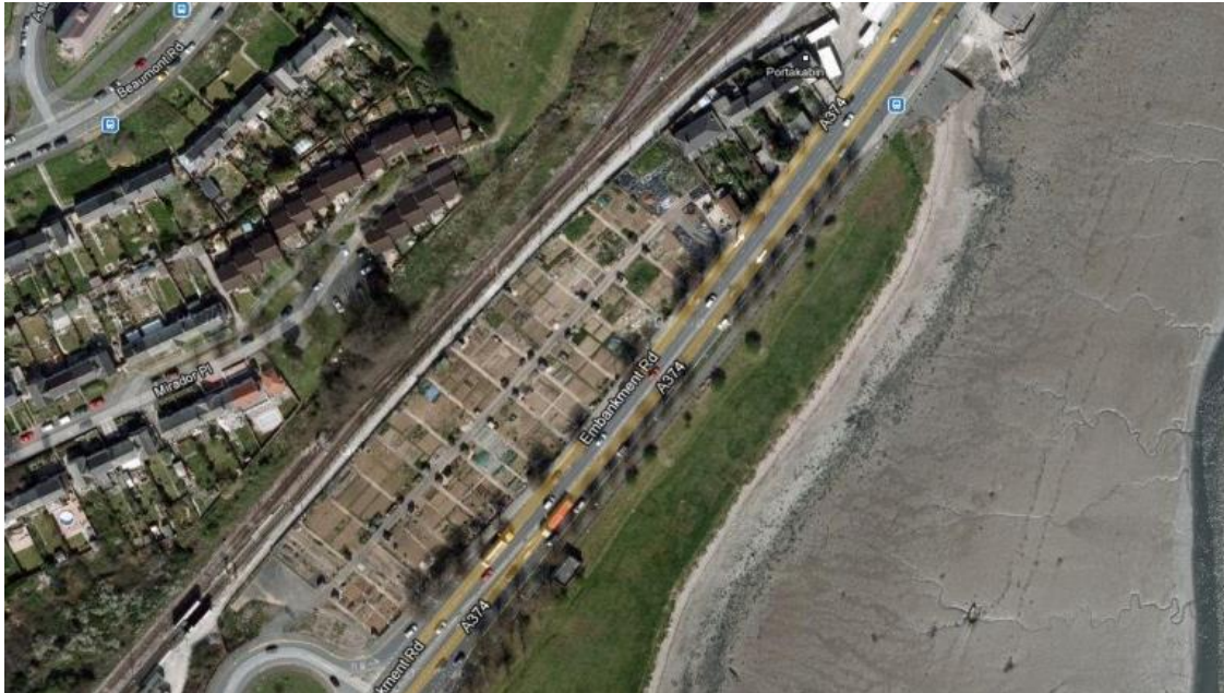
Figure 4.9(c) Embankment Road
