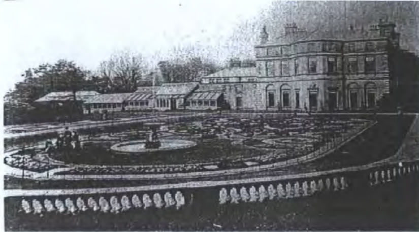
57. The Formal Garden at Worden Hall, Lancashire.
