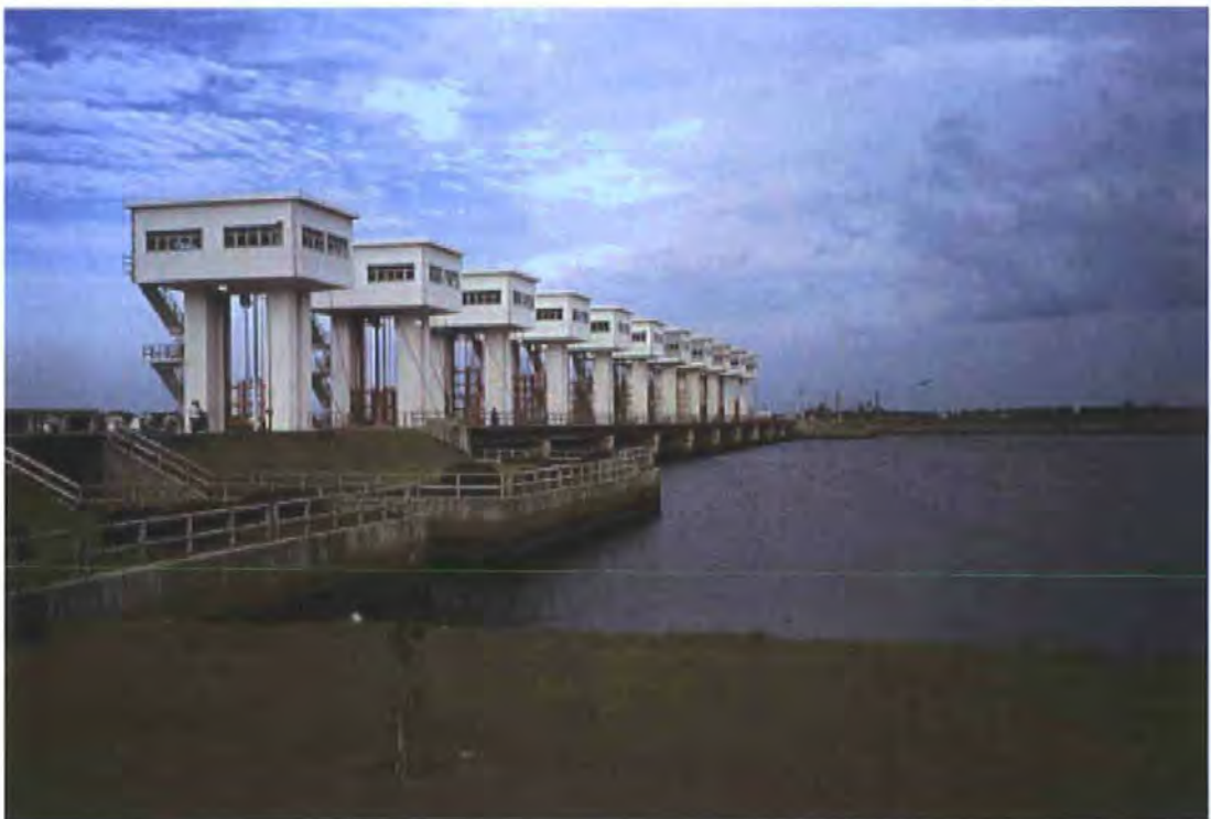
Figure 3-4 The Pak Pa-Nang River Barrier (opened in September 1999).
