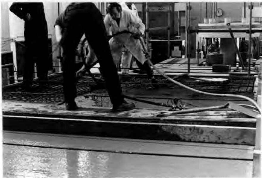
Figure 8.9: First deck under construction
