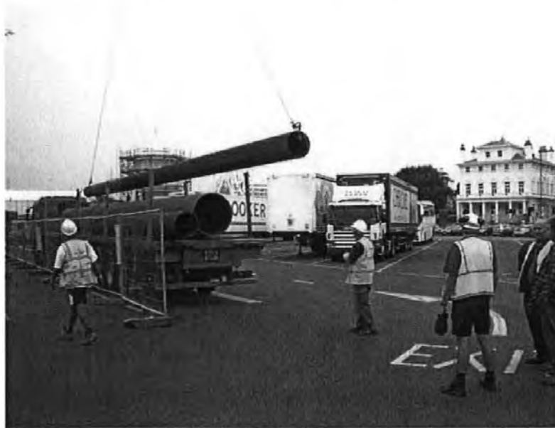
Figure 7. Photograph of pile tubes being unloaded.
