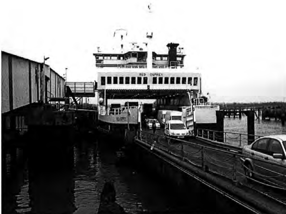
Figure 1. Photograph taken from quayside with ferry docked at terminal, and vehicles disembarking along linkspan. Structure on left of photograph is covered walkway for pedestrian passengers, and the dolphin on which it rests can be seen.
