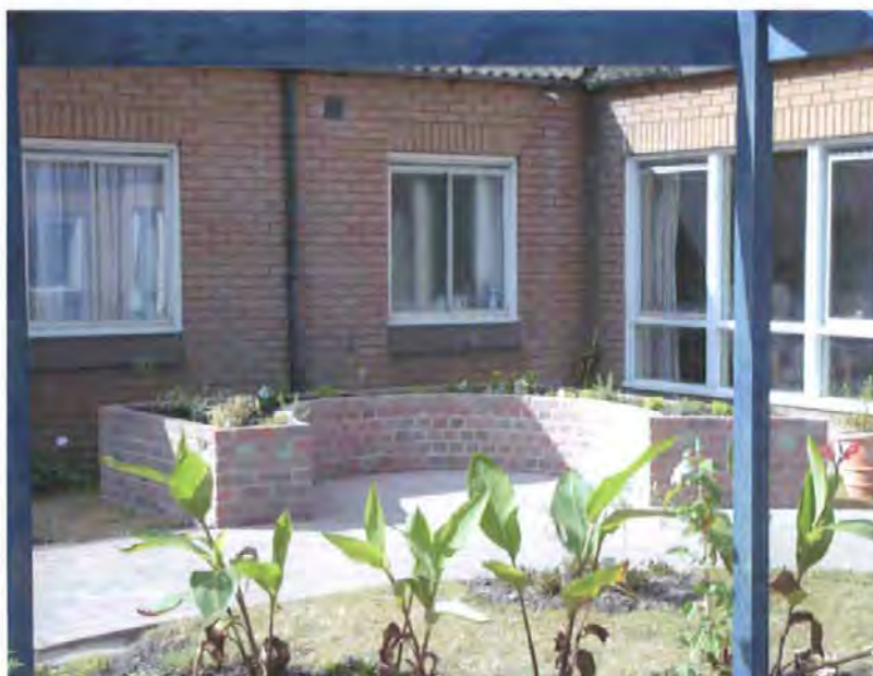
Brick raised bed after top layer had been removed
